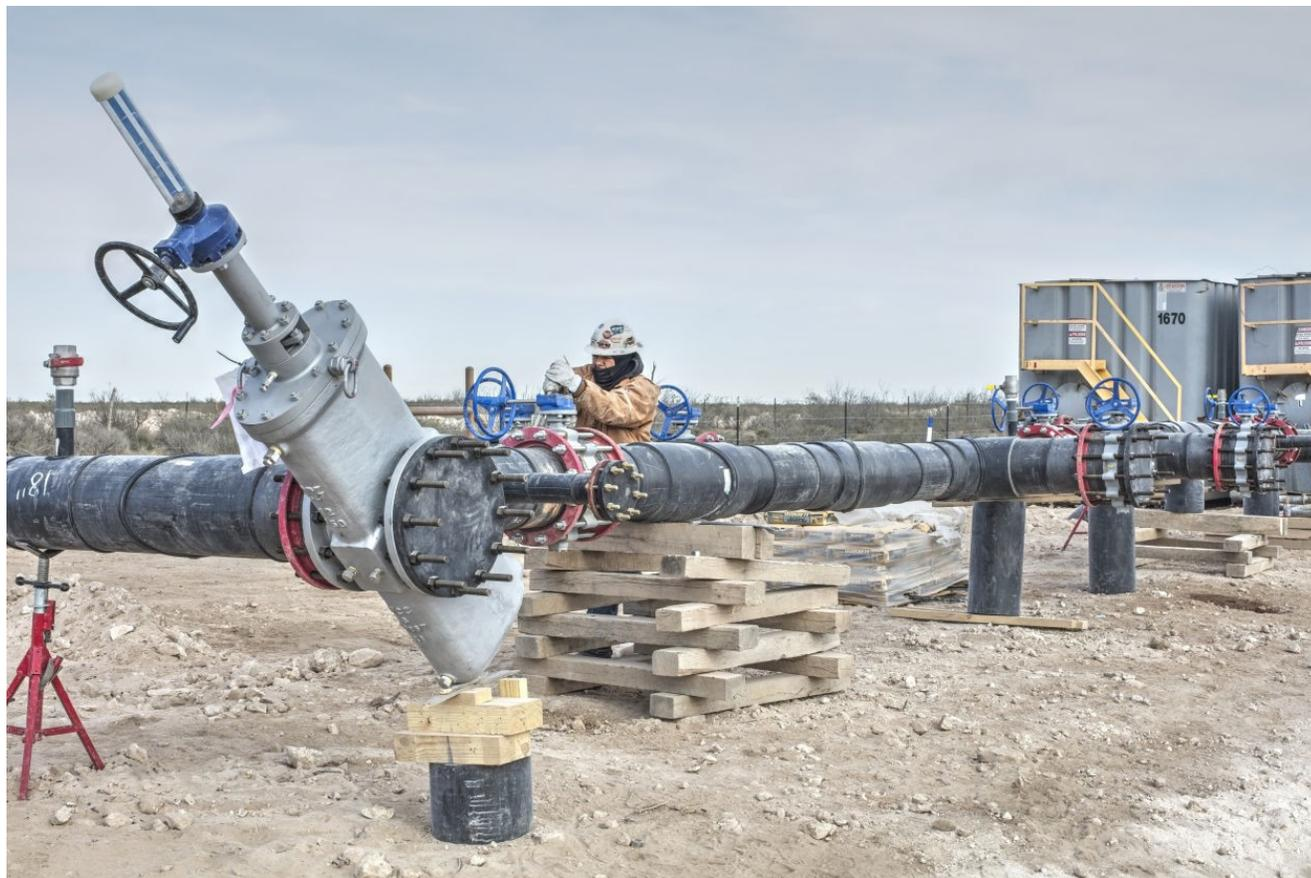
A worker installs a valve station at a WaterBridge Resources wastewater handling system in West Texas.
